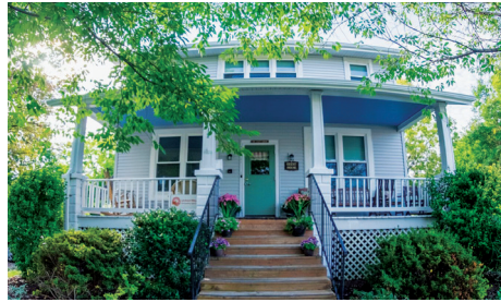
After much needed repairs and renovations to the Guest House.
