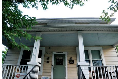
The Guest House in need of repairs.
