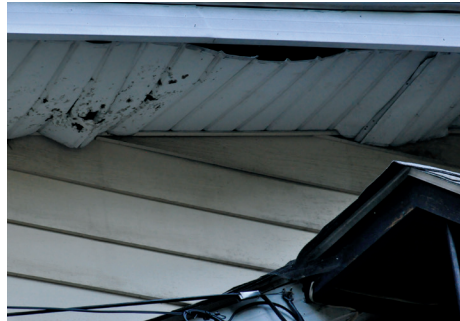
Signs of much needed repair at the Guest House.
